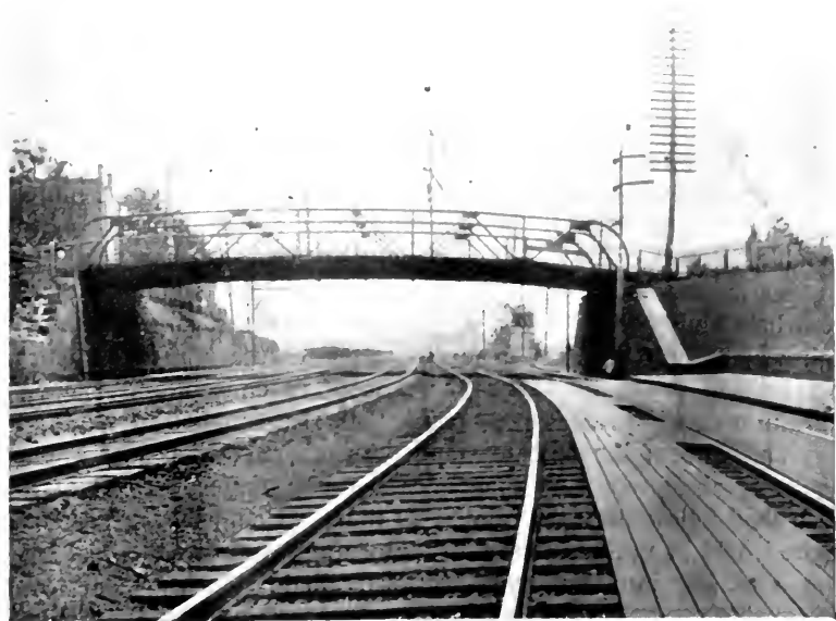
A HIGHWAY BRIDGE USED FOR CARRYING OVERHEAD SIGNALS.
